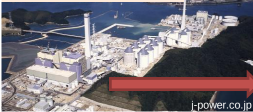
Coal power generation
