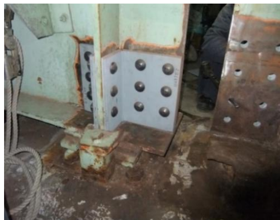
Application examples of focused repair method
