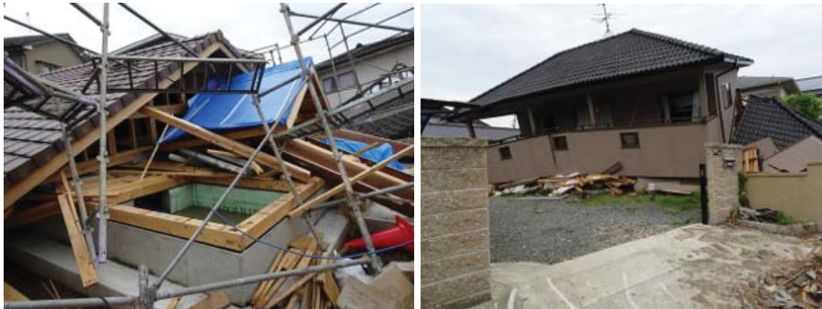
Photo. Damage of the dwellings caused by the Kumamoto earthquake in Mashiki Town
