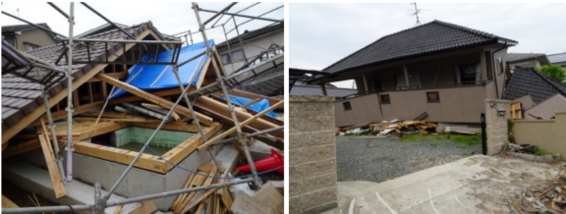
Photo. Damage of the dwellings caused by the Kumamoto earthquake in Mashiki Town
